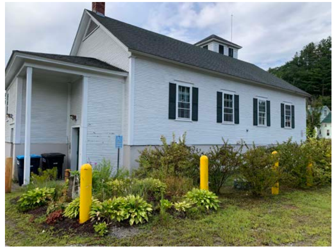
Back of building (no handicapped parking) Handicapped entrance door to left of HC parking sign
